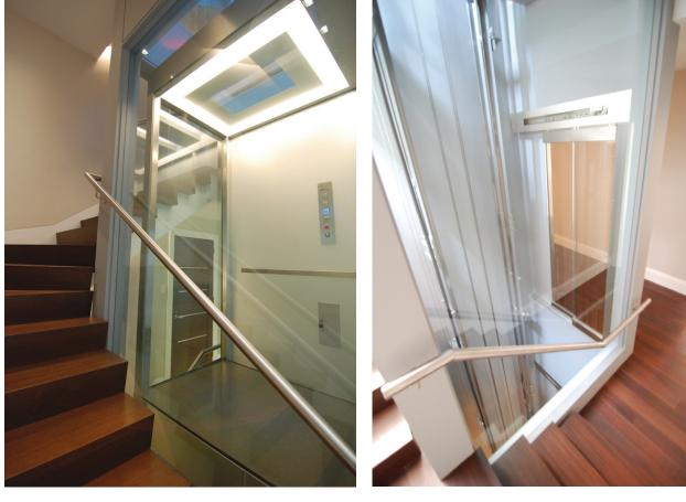
"The counterweights served as a moving backdrop for people on other floors to view as the elevator was in motion. The cover for the counterweights was powder coated a different shade of gray with more of a sheen/sparkle differentiation from the other structural components."
