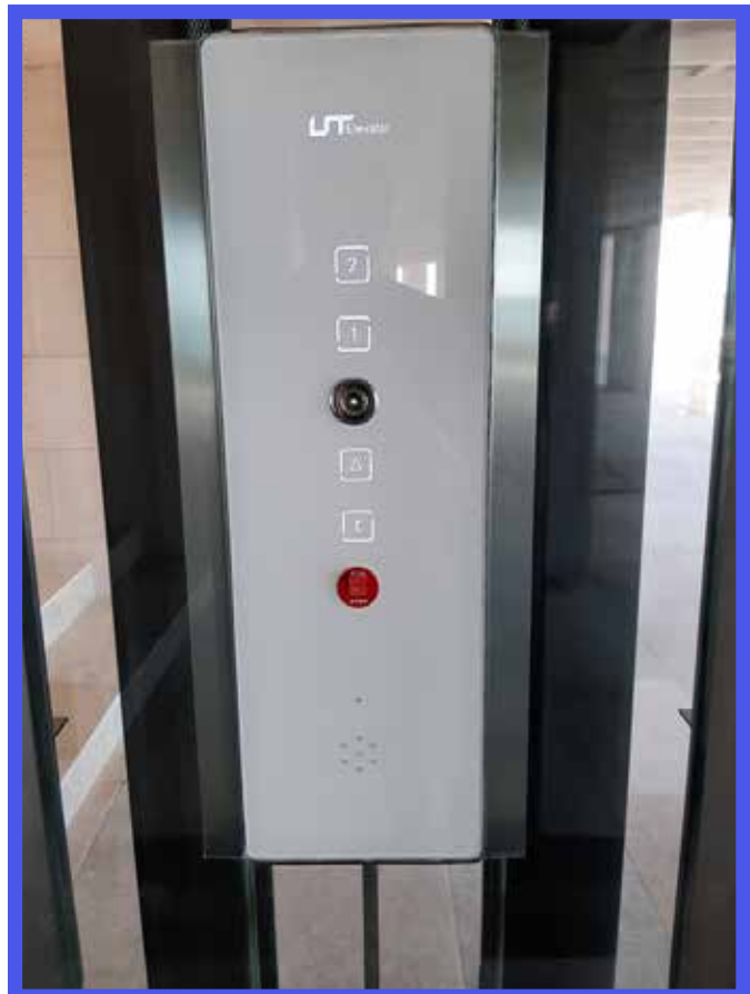
Capacitive-touch glass fixtures were embedded into the control side glass panel for a uniform, flush appearance.
